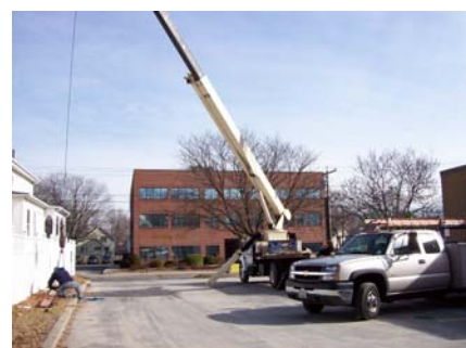
A crane was used to lift steel beams into the building.
